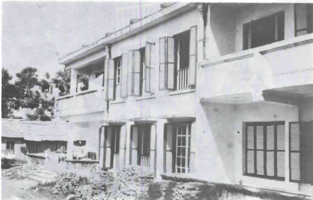
Plate 6. The existing two-storey building.
